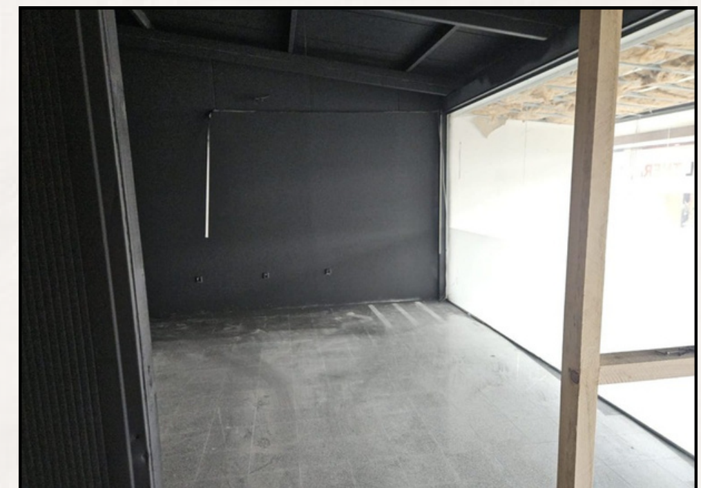
Shell construction – Space II
