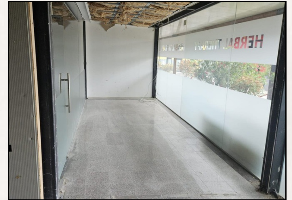
Shell construction – Space I
